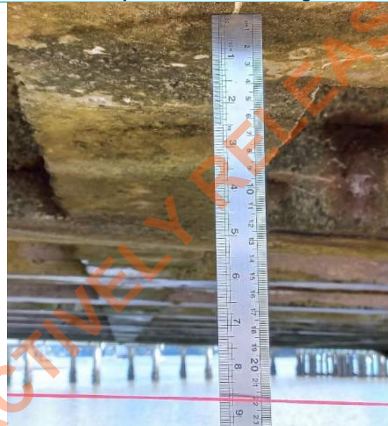
2023 inspection reading at the southeast outer girder = 220mm
