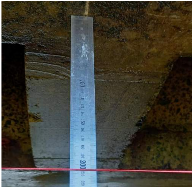
2021 inspection reading at the northeast outer girder = 205mm
