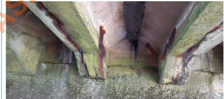
15mm- 22mm significant Longitudinal concrete cracks along existing P.C beams with severe induced corrosion of reinforcement bars.
